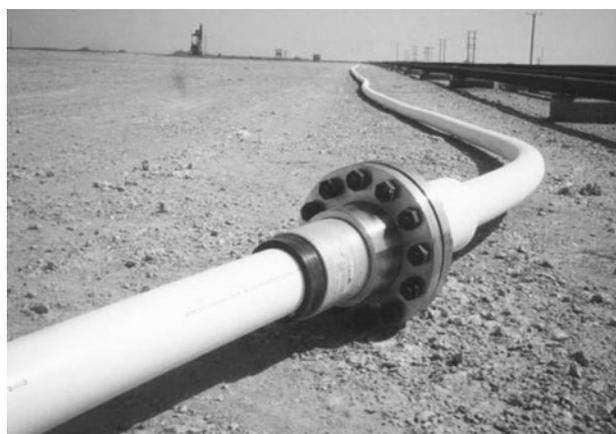
3 Aramid fibre RTP in use for transport of oilfield fluids: photograph shows white pigmented, UV stabilised cover for exposed use in hot climates, as well as electrofusion coupler technology, which is one of jointing options (Courtesy Pipelife bv)
